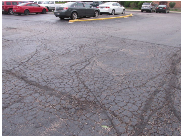
Alligator cracks adjacent to recent patch repair
