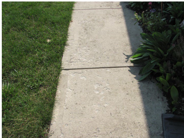
Spalled concrete sidewalk at Unit 200
