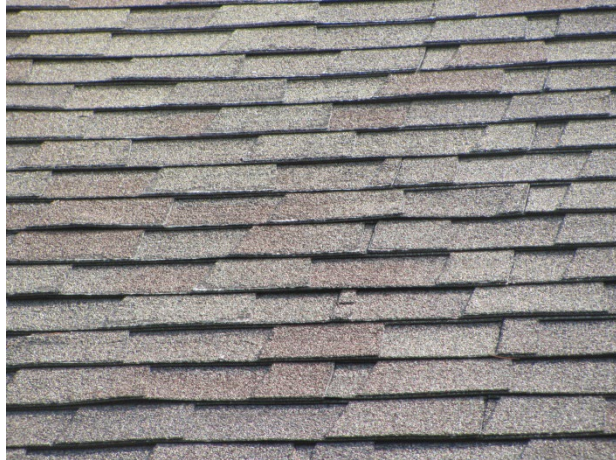
Granular loss evident at shingles at Unit 600
