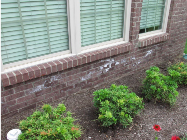
Efflorescence and evidence of water infiltration at Unit 100
