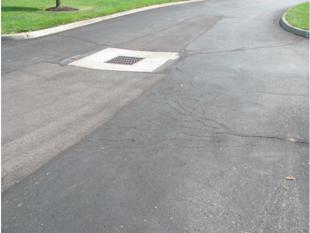
Recent asphalt pavement repairs near community entrance
