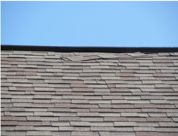
Loose shingles at Unit 100
