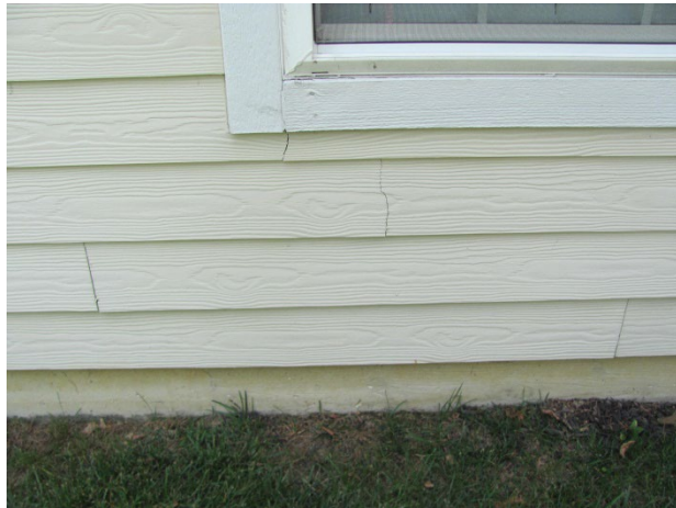
Isolated fiber cement cracks at Unit 500
