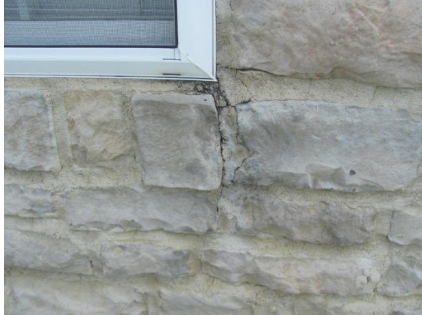
Mortar deterioration at Unit 200
