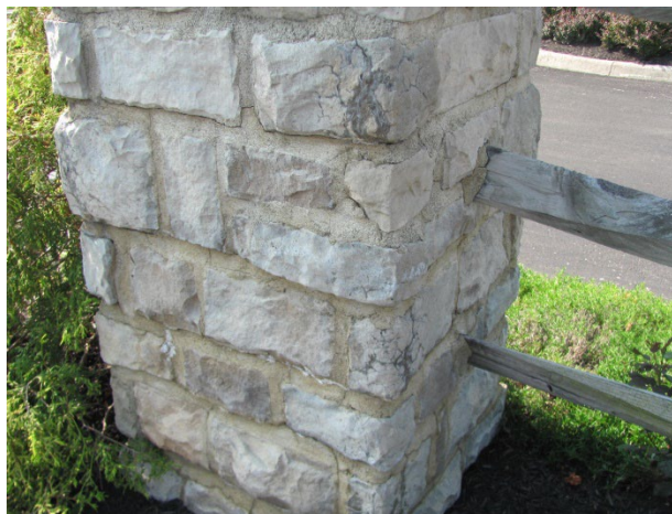
Evidence of water infiltration and possible onset of stone delamination
