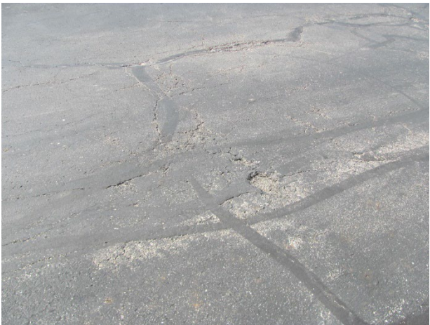
Pavement raveling and onset of potholes
