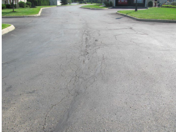
Centerline cracks and deterioration
