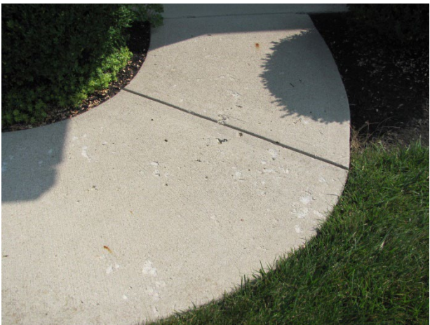
Spalled concrete sidewalk at Unit 100
