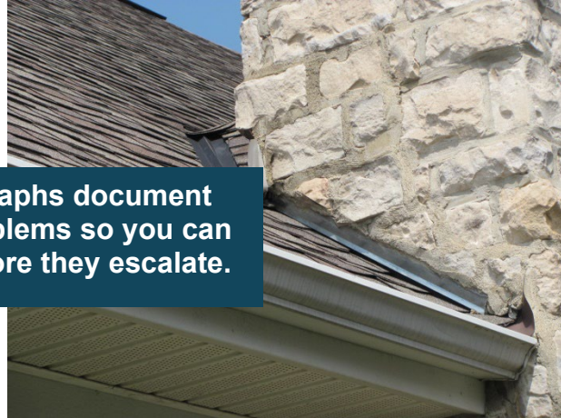
Flashing detail at chimney
