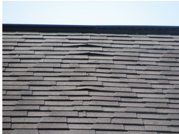
Lifted shingles at Units 200 and 201
