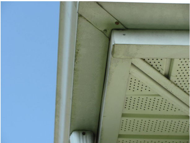
Fastener rust evident
