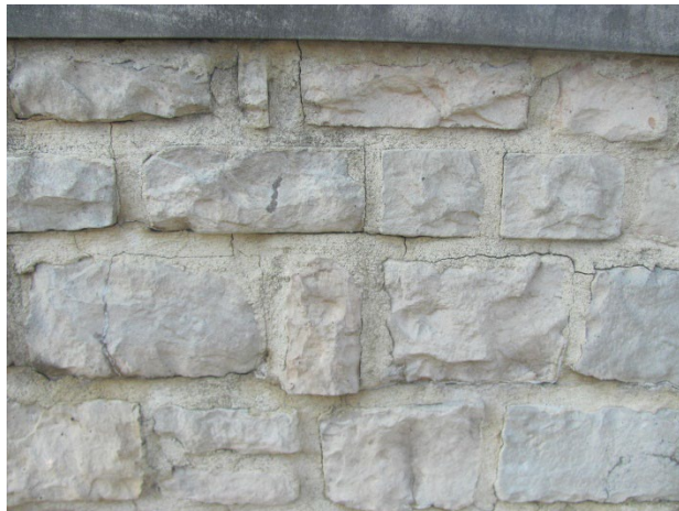
Mortar cracks
