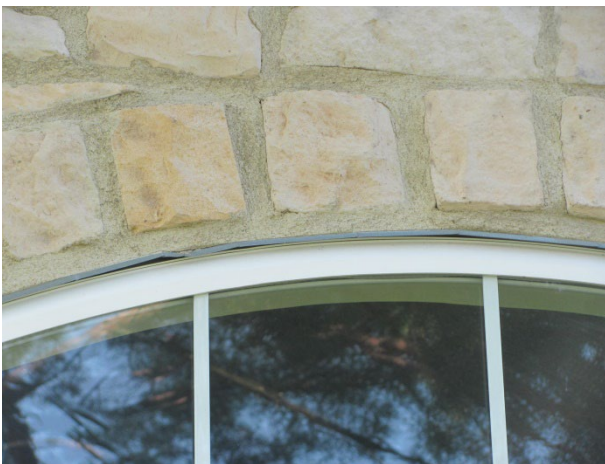
Flashing detail above window
