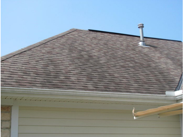
Weathered shingles at Unit 500
