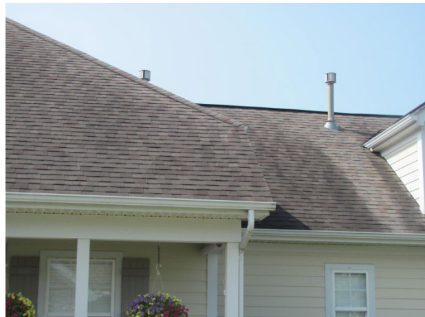
Weathered shingles at Unit 400
