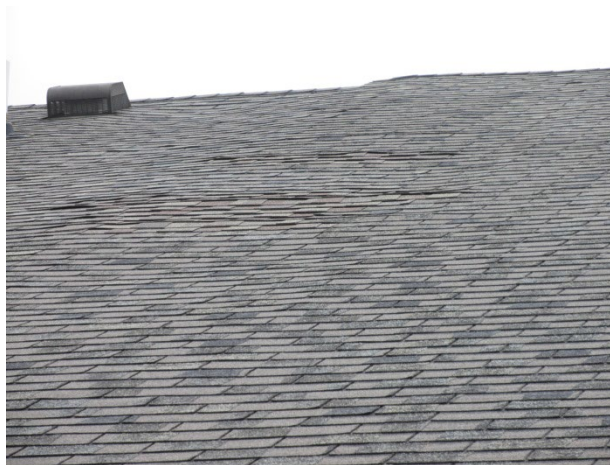
Sheathing deflection evident at Unit 700
