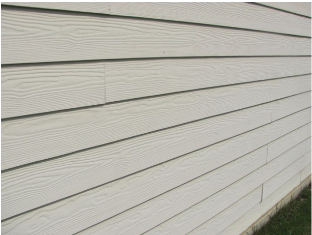
Fiber cement siding
