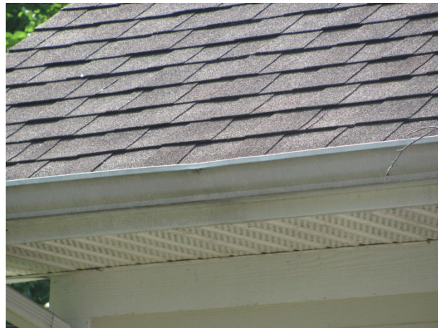
Minor dented aluminum gutter section
