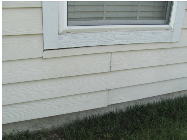
Isolated fiber cement crack at Unit 700
