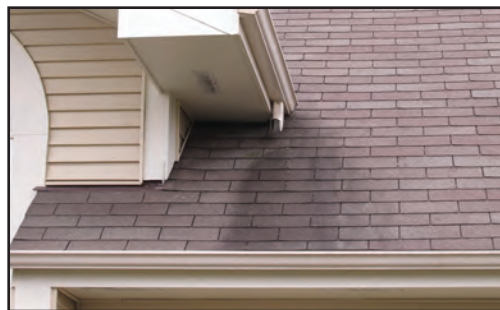
Downspout discharge directly onto shingles
