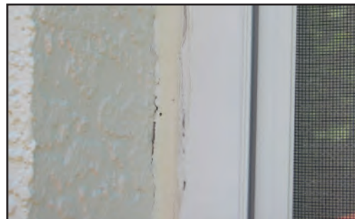
Sealant adhesion failure
