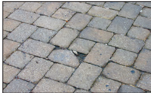
Paver damage
