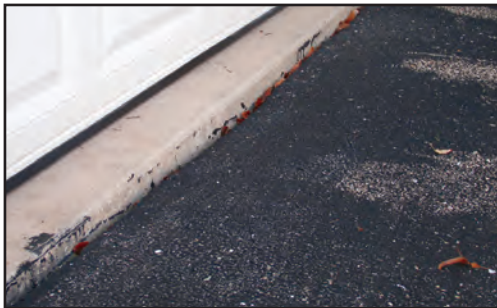
Settlement at garage threshold
