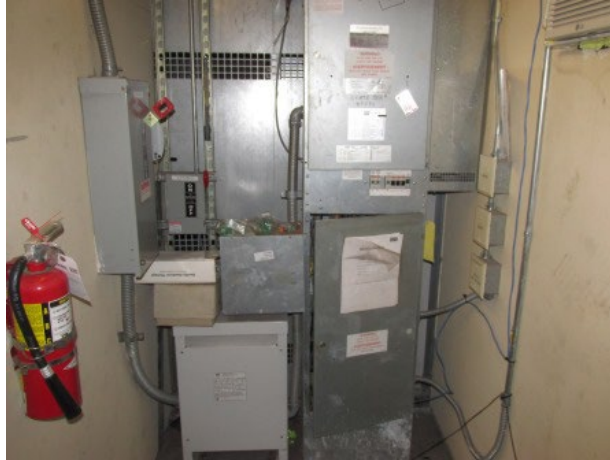
Machine roomless elevator controls
