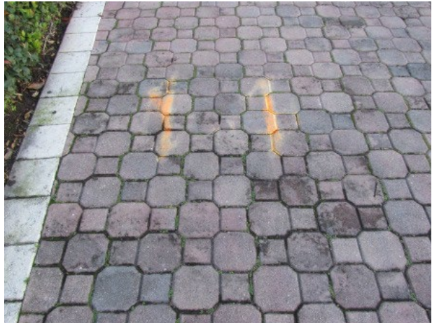
Displaced and settled pavers
