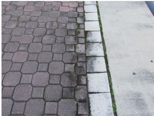
Displaced and settled pavers
