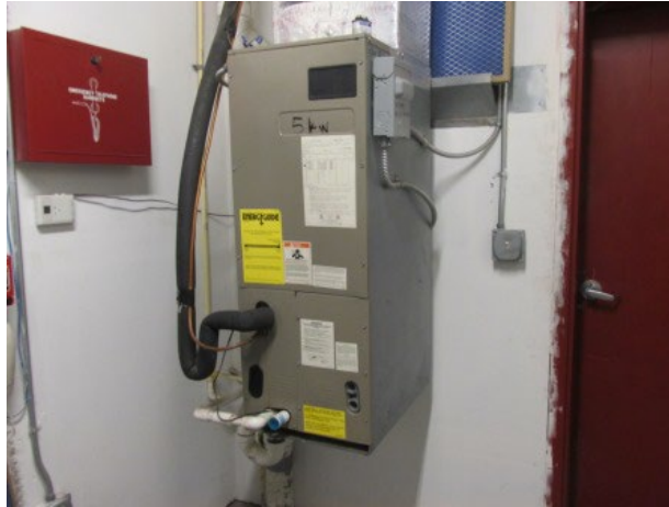
Typical interior air handling unit
