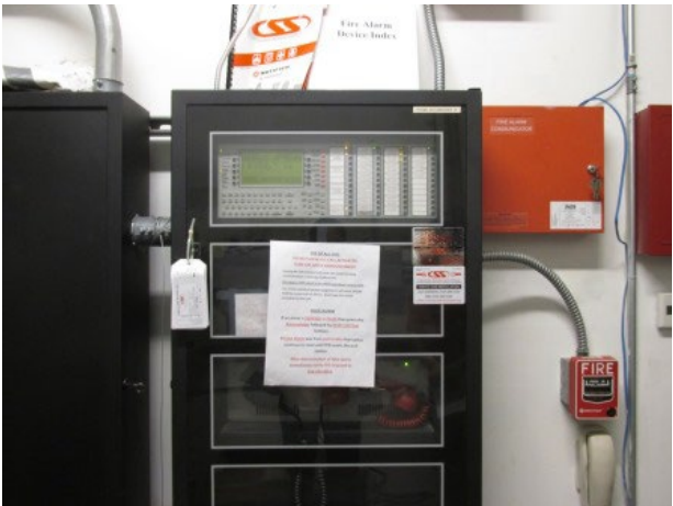
Life safety system control panel
