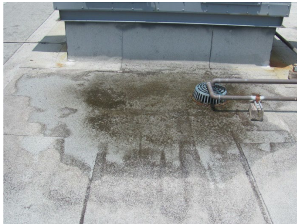
Modified bitumen roof – ponding at drain
