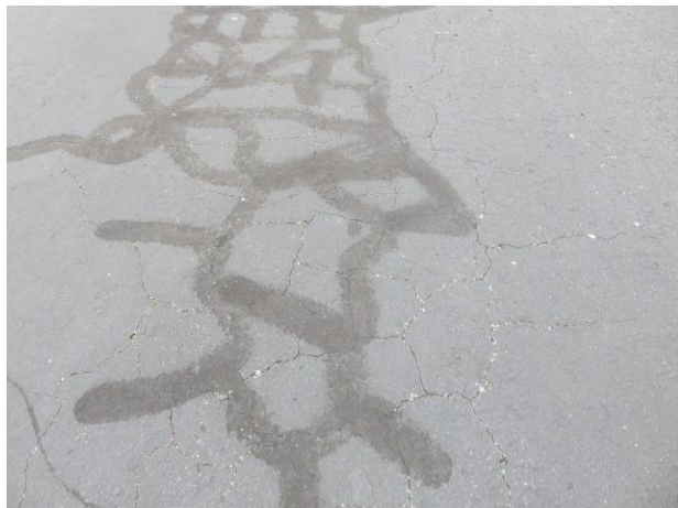
High frequency of cracks
