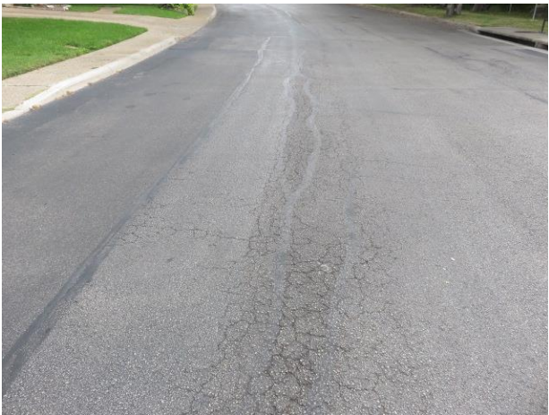
Alligator cracks
