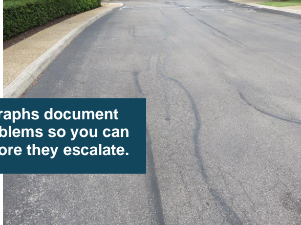
Alligator cracks
