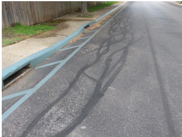
Repaired edge cracks
