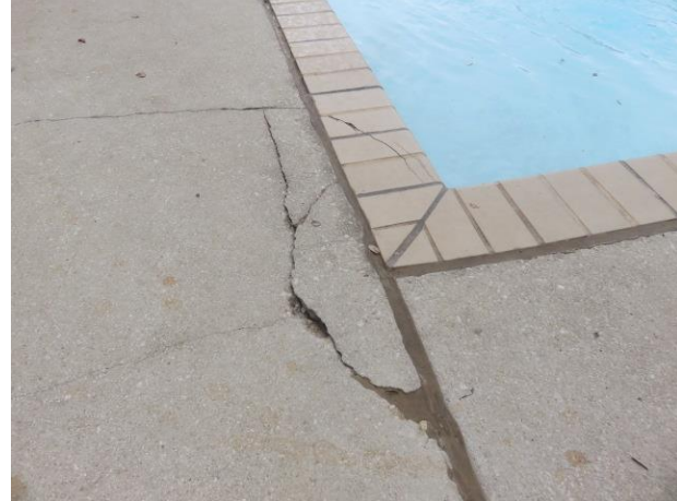
Significant pool deck cracks
