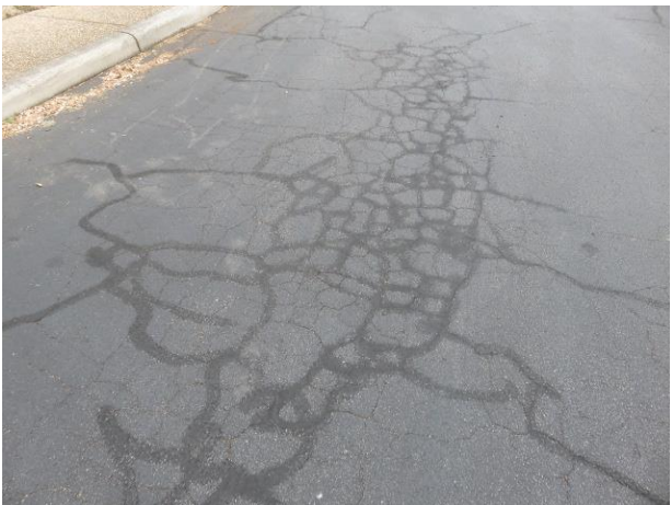
High frequency of cracks
