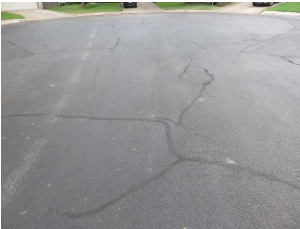
Crack repairs at cul-de-sac
