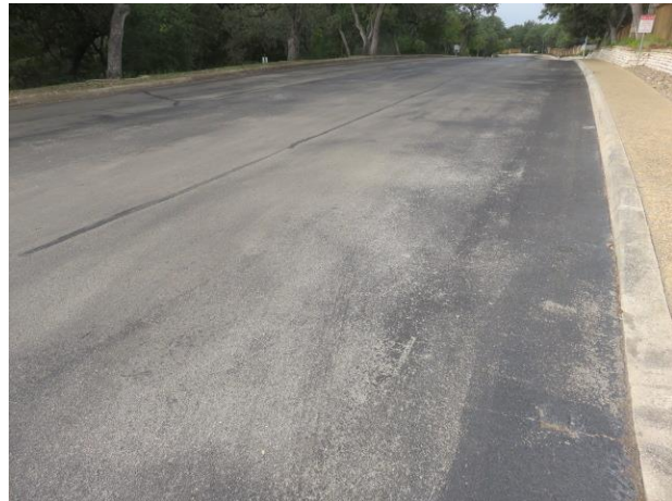
Repaired longitudinal cracks at centerline and edges
