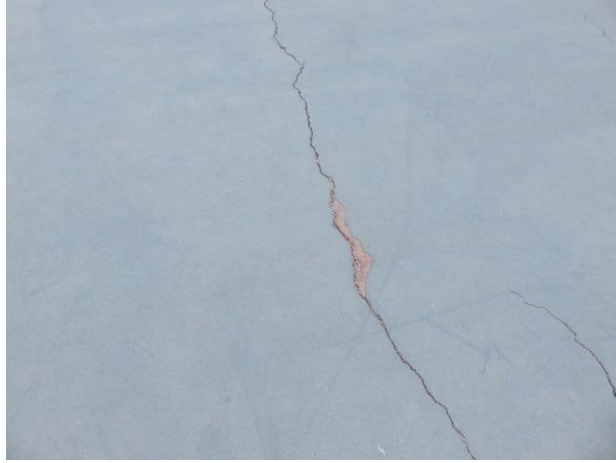
Wide cracks at tennis court
