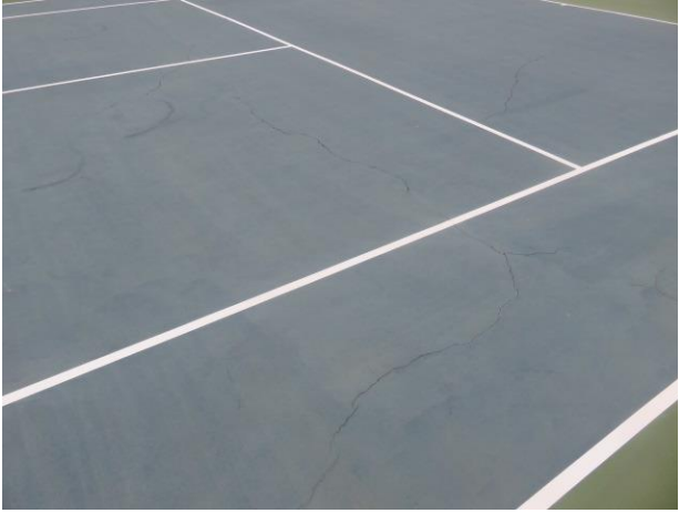
Cracks at tennis court playing surface
