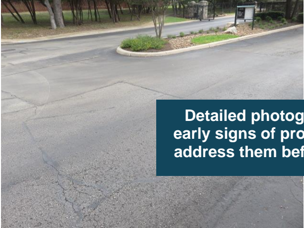
Repaired and unrepaired cracks near gates
