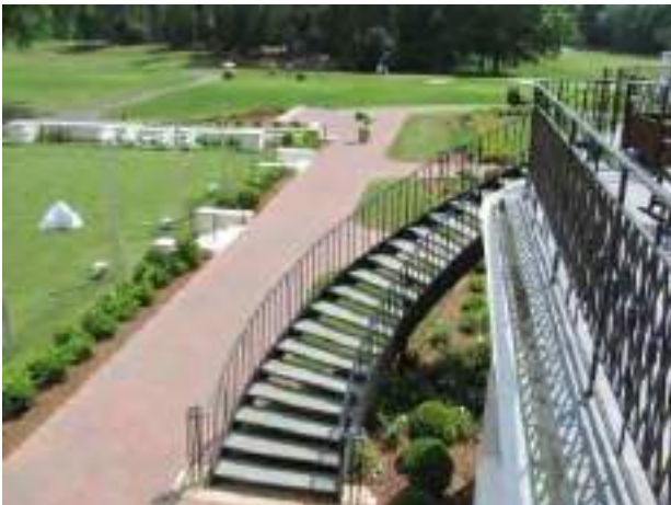
Metal and concrete staircase at clubhouse
